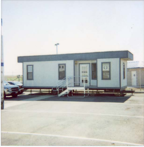
LOOKING SOUTH (NORTH SIDE)
